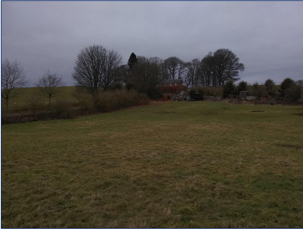
Plate 2: North-west facing view of the Category C Listed Kemphill Farmhouse (Site 15)
